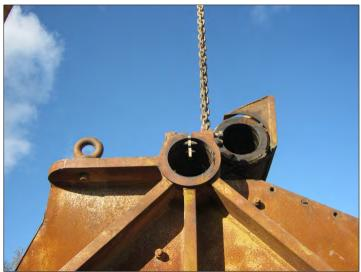
Work Starts Striping out hinge pin and eccentric shaft
